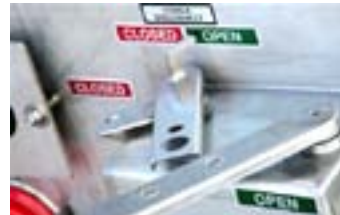
Interlocking Handles: Visible Disconnect & Load Break Switch or VFI
