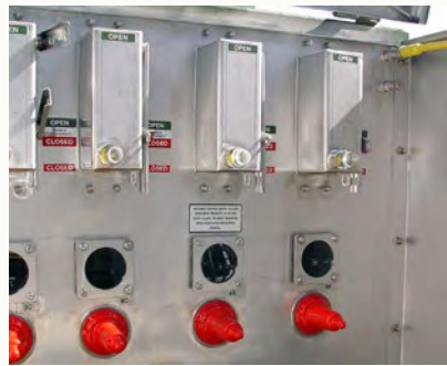
Single-Phase Visible Disconnects Switches
