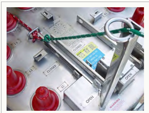
360° Open Rope Operator with Upper Stanchion Ring
