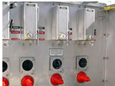
Single Phase Visible Disconnects Switches
